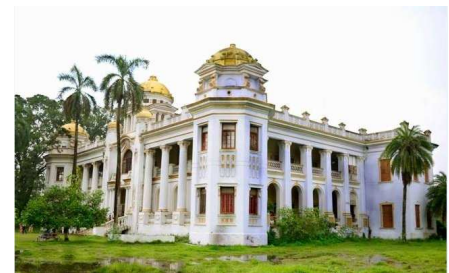
View from south-west corner
